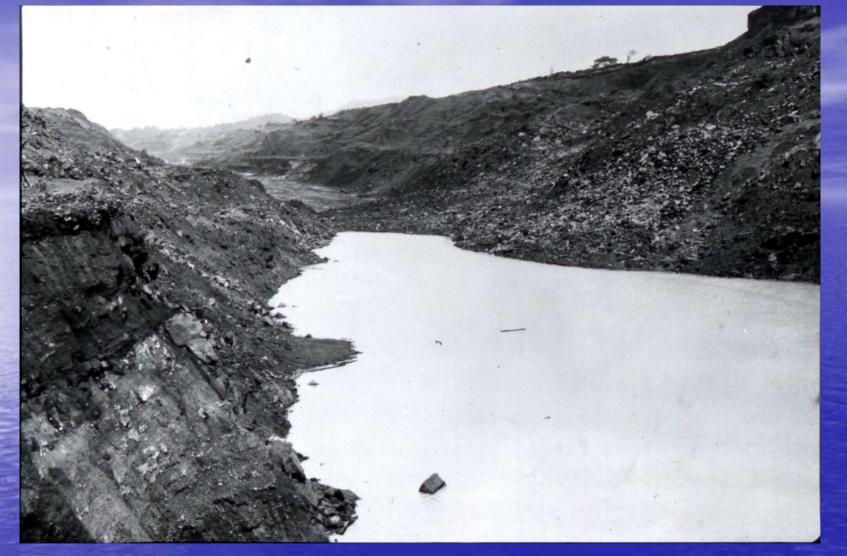
Landslides began to plague the French excavations in the vicinity of Cucaracha and Culebra in 1886, severing their trunk rail lines. In addition to slides, they fought a losing battle with Yellow Fever and Malaria, and went bankrupt in 1889.
