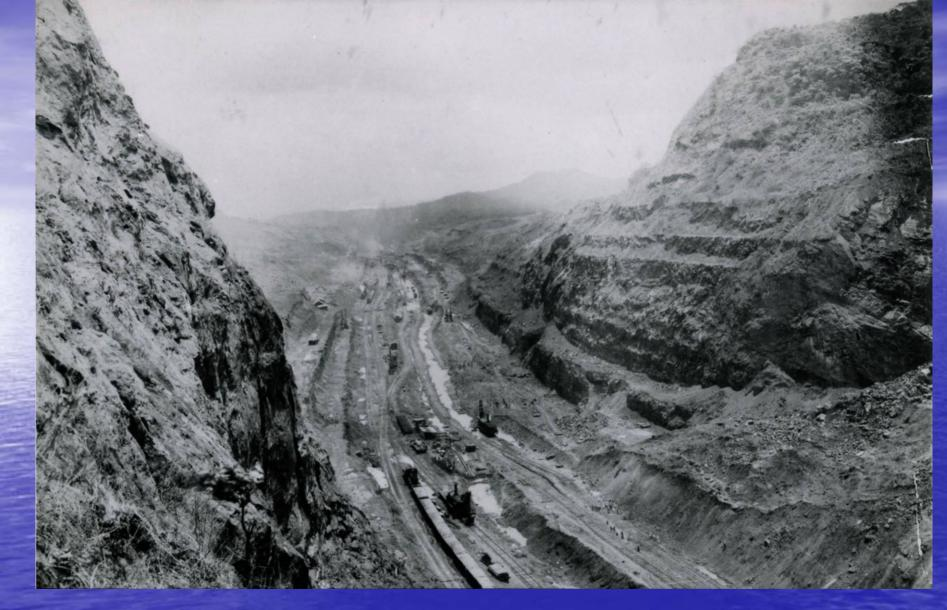
Closing in on the finish line. Looking into the gapping hole at the Continental Divide on May 17, 1913. Note 1/2:1 side slopes.
