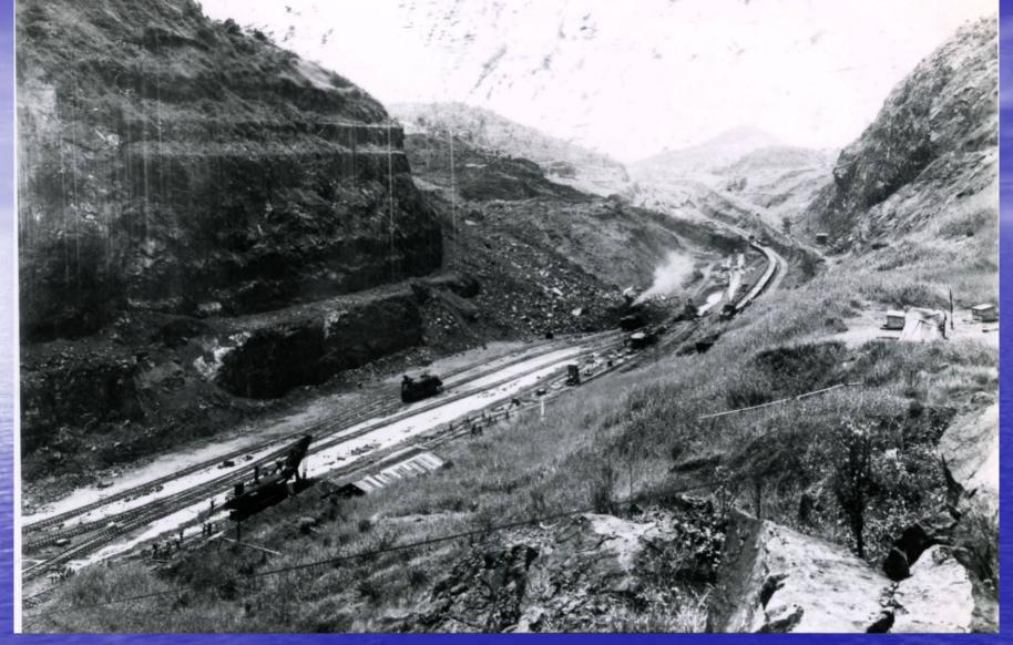
Excavating debris at the toe in the wake of the first massive slide at Cucaracha, on August 20, 1913.
