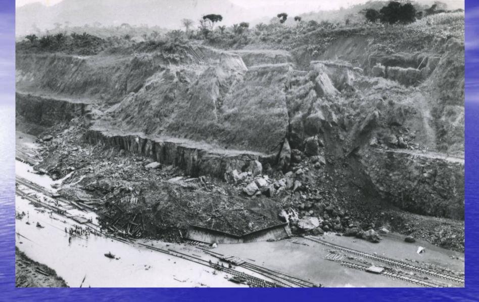
Cut slope failure on the Obispo Division on August 21, 1912. Note ponded water.
