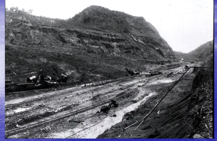
As the excavation deepens, the side slopes started caving in on the main excavation. This shows the beginning of the East Culebra side
