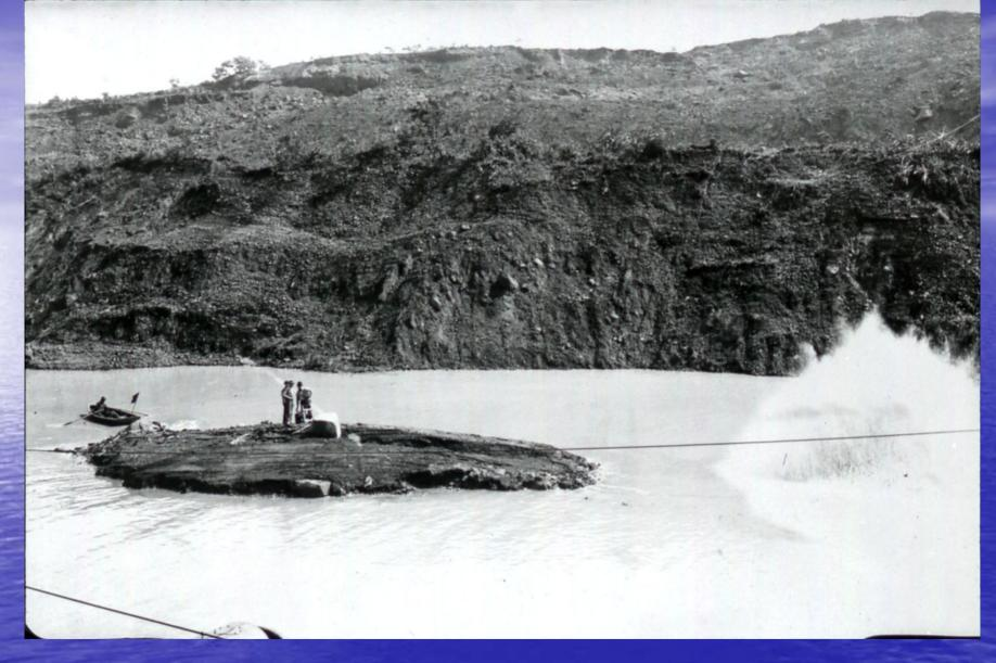
Toe heave that protruded upward through 30 feet of water on September 19, 1915.
