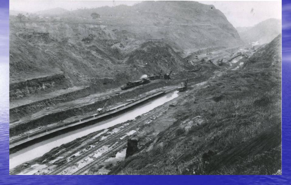
Large deep-seated slump on the East Culebra Slide blocks the canal excavation, May 27, 1913.
