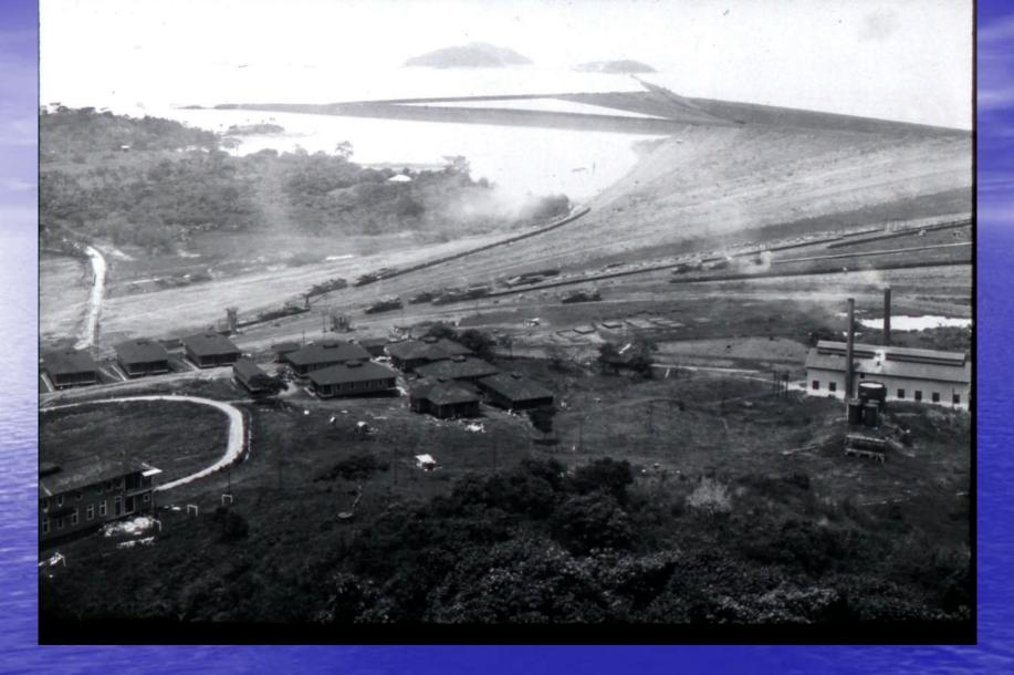
The waste muck was conveyed by rail cars and dumped into enormous fill piles at the coasts.
