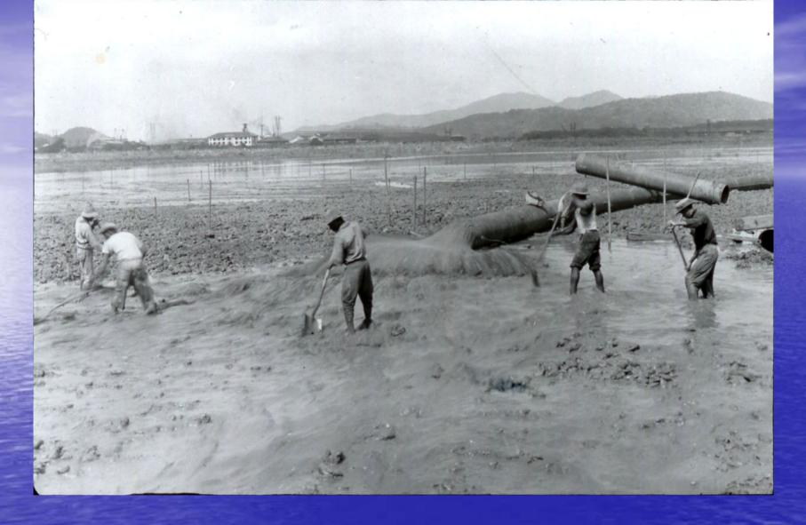
Outfall discharge from a suction dredge. The dredge tailings were dumped into rock-lined dikes.
