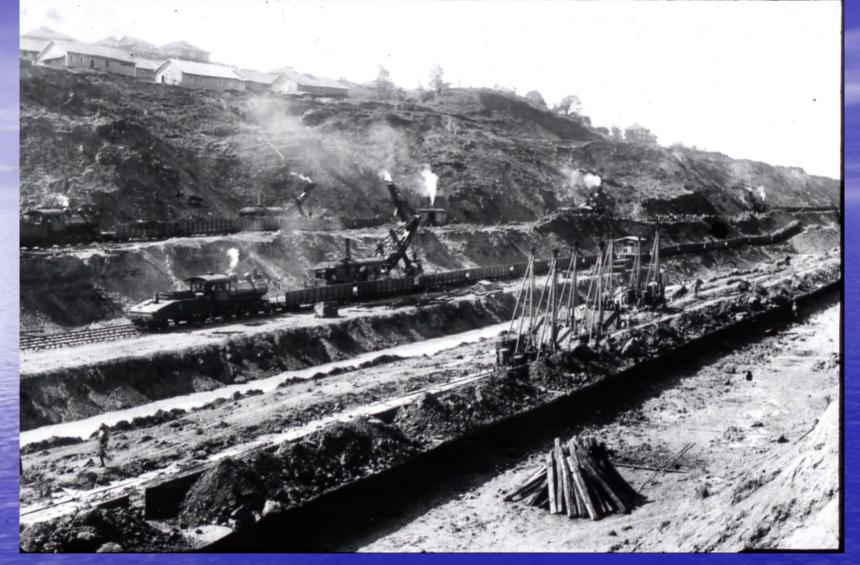
Legendary railroad engineer John F. Stevens conceived a plan to construct a locked canal, using water from the Chagres River to create a vast inland lake. This reduced the required depth of excavations by 70 feet.
