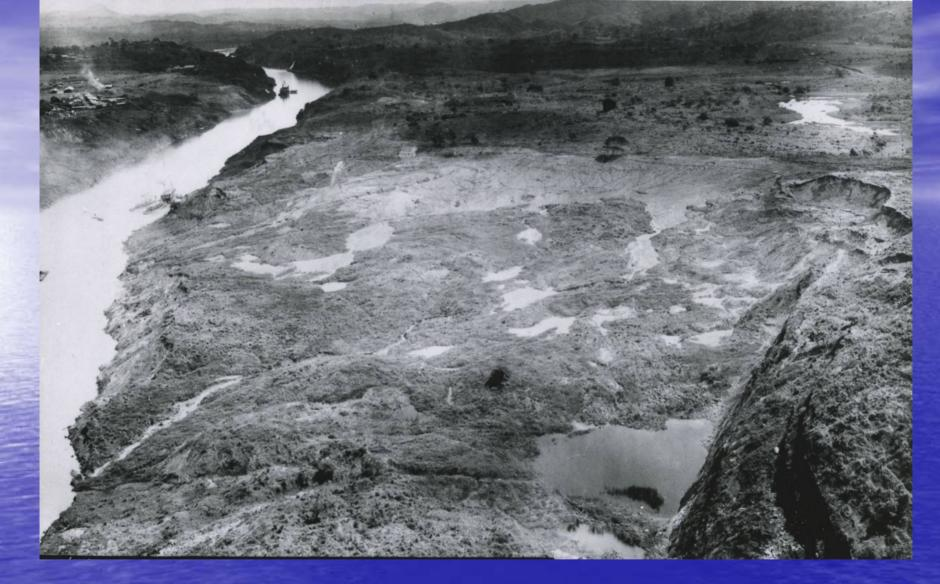
East Culebra Slide as seen from the crest of Gold Hill on June 19, 1923. The shear strength of the slide debris had obviously been transformed to a much lower value.
