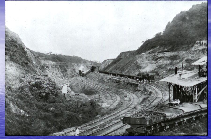
The 45 degree side slopes of the massive cuts can be appreciated in this view, as the Americans begin to attack the Continental Divide.
