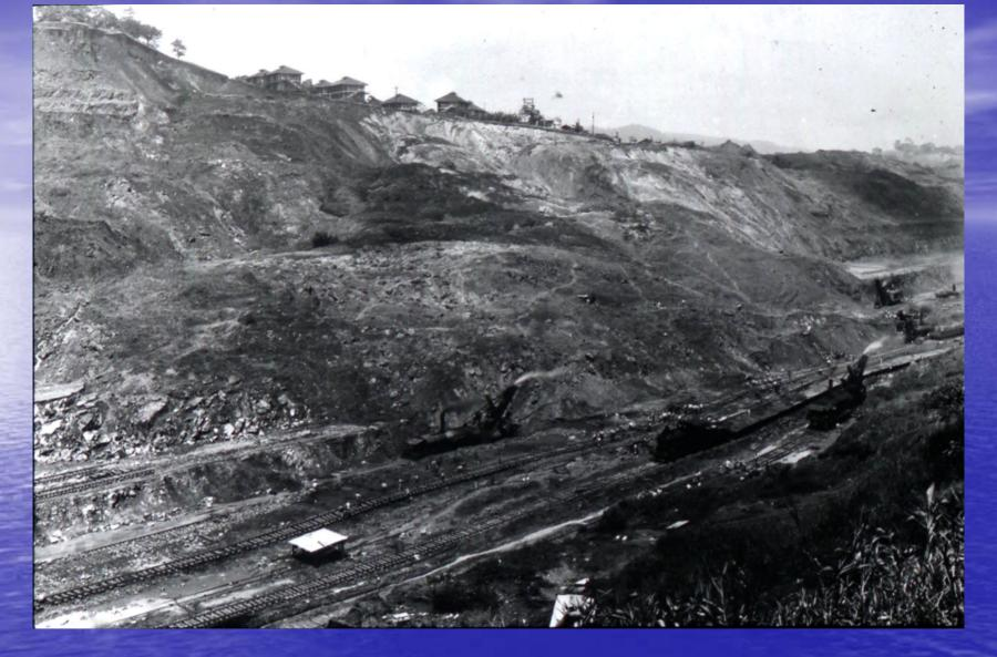
Excavating the toe of the West Culebra slide with steam shovels, and allowing the slide debris to disintegrate and slide into the hole.
